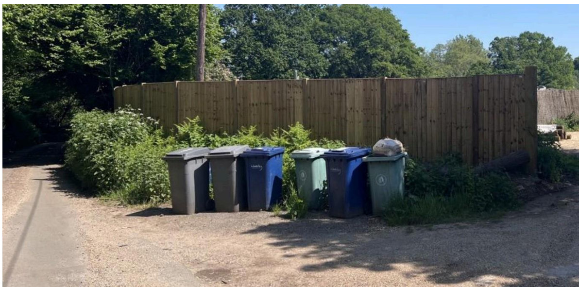
Figure 3: Illegal closeboard fencing too high alongside the public highway of Thorncombe Street.
