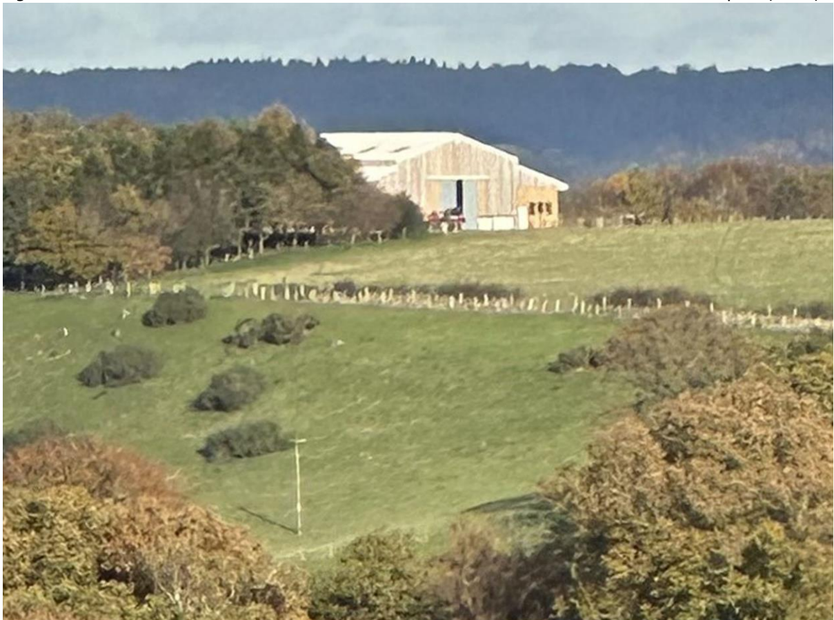
Figure 4: Further 'works' to the barn as it stands to date - 2024
