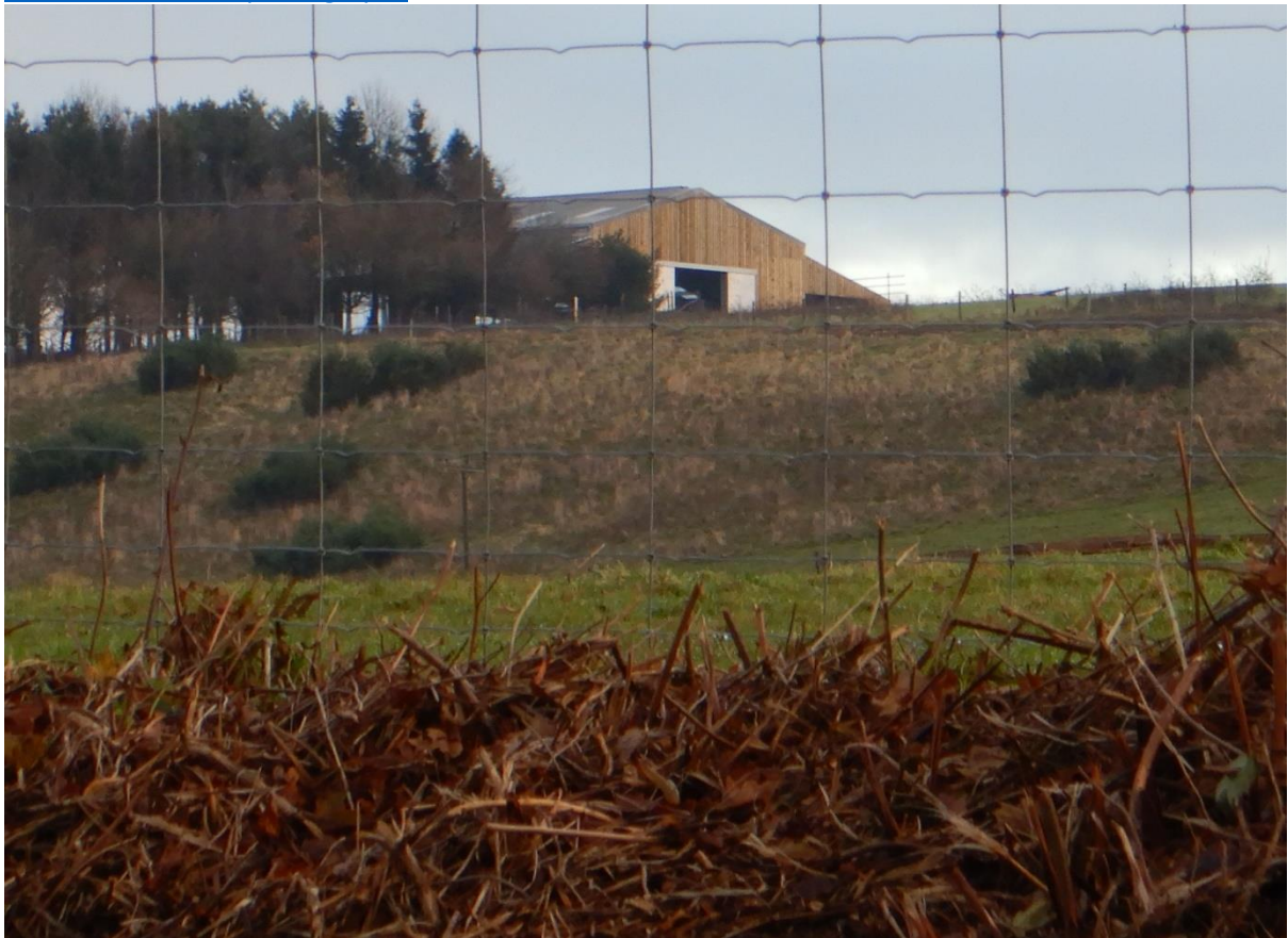
Figure 3: As Built barn with aisles either side and not in the location shown on the block plan (2021).
