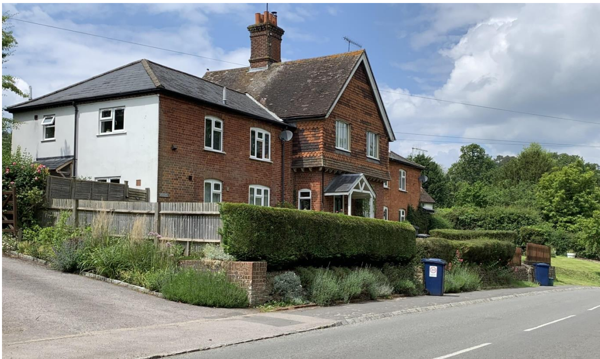
Figure 1: No 3 Millpond Cottages, The Street, Hascombe showing the terrace of cottages set high on the bank, fronted with a Bargate stone retaining wall.
